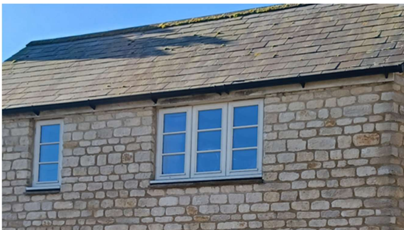
Fig.30: Limestone and grey slate roofing, casement windows in new build
