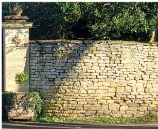
Fig. 25 Drystone walling, stone coping
