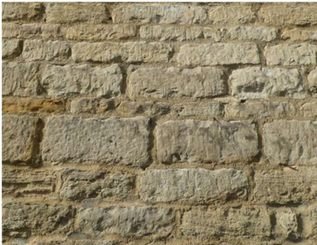
Fig. 28 Squared, coursed limestone
