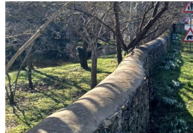
Fig.27 Cement mortar capping
