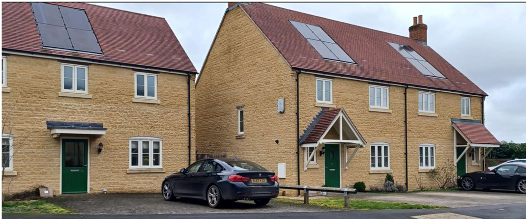
Fig. 33: C21 housing with solar panels, Marriott Close
