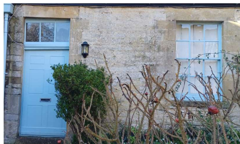
Fig. 21 Panelled door and 6/6 sash
