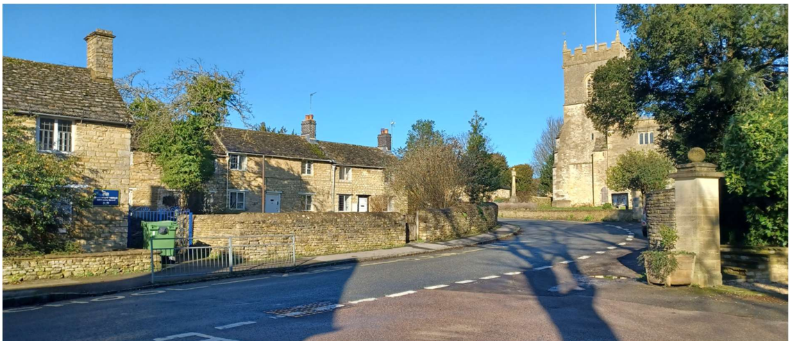
Fig. 3: Parrotts School, School Cottages and St Mary's Church, Church Street
