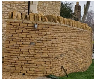
Fig. 26: Drystone walling, stone on edge capping
